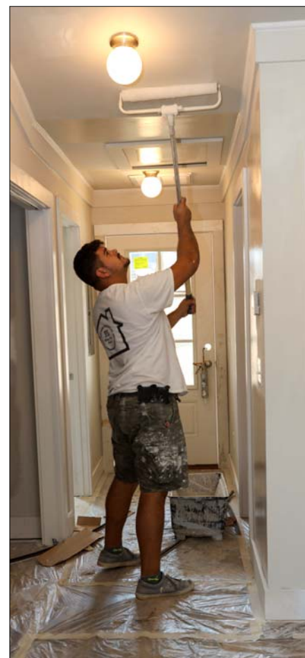
Home repairs program at work
